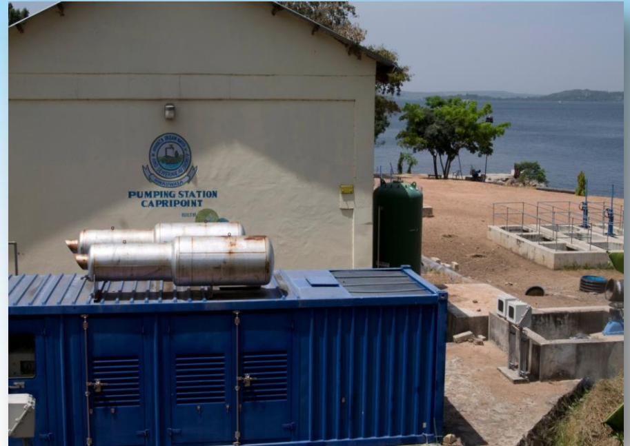
Capri-Point Water Intake and Pumping Station
