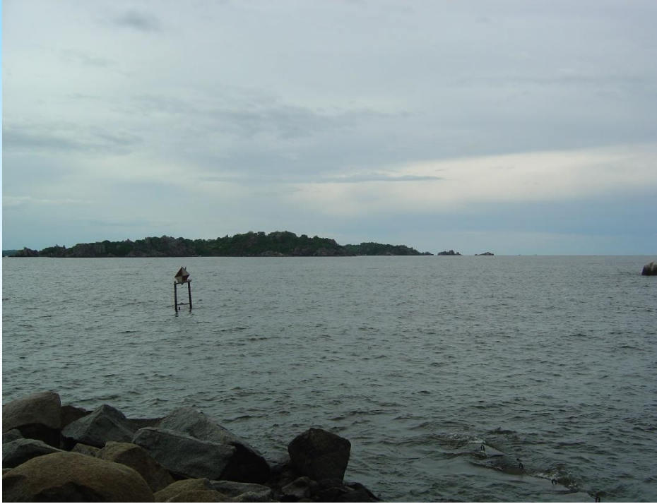
Mwauwasa abstraction point at Capripoint water intake.
